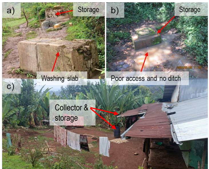
Figure 3 Protected springs with a) large storage capacity, a separate washing slab and good accessibility and b) poor condition with limited storage, a submerged outlet in polluted water and difficult access. c) Rooftop with collection gutters and a small container for storage.
